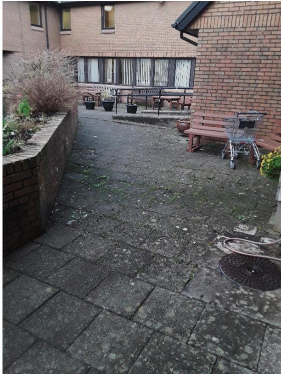
Photos of before and after work at Dunmar Court, Oban
